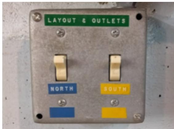
To turn on power, both switches must be flipped up. It is important that they both be in the same position. When turning on power, please also turn on all the lights, including the switch to the left of the “Layout & Outlet” Power.
